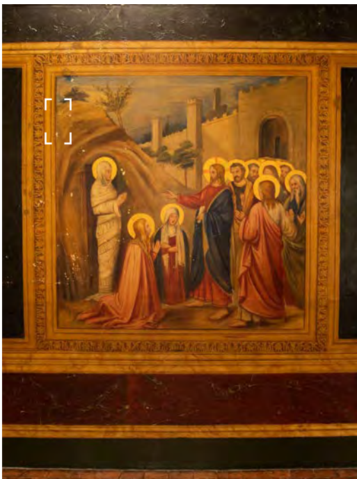
Fig.10 Detail of the east wall where blistering and flaking paint is concentrated. It would appear this is due to a localised cause. Possibly water infiltration.
