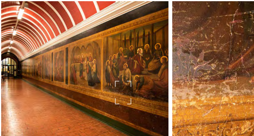
Fig.4 View of the north corridor where damage from passers-by is most evident.
